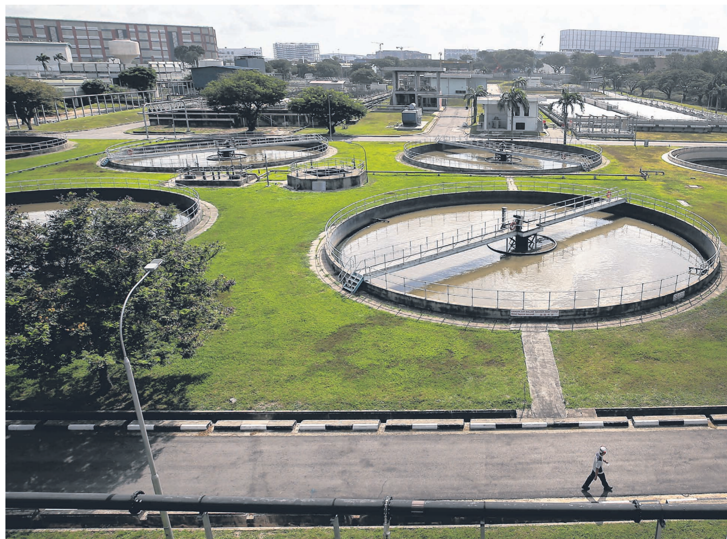
Circular sedimentation tanks are a distinctive feature in the landscape of Jurong Water Reclamation Plant. Jurong WRP, in operation since 1981, will be phased out by 2025 when the DTSS Phase 2 project is completed.
