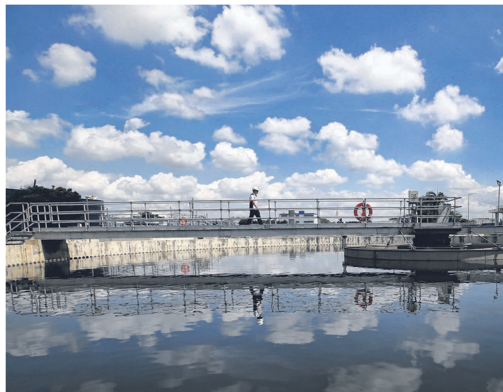
Above: Treated used water, or secondary effluent, at Jurong Water Reclamation Plant, is channelled through effluent outfall facilities for discharge to the sea.
